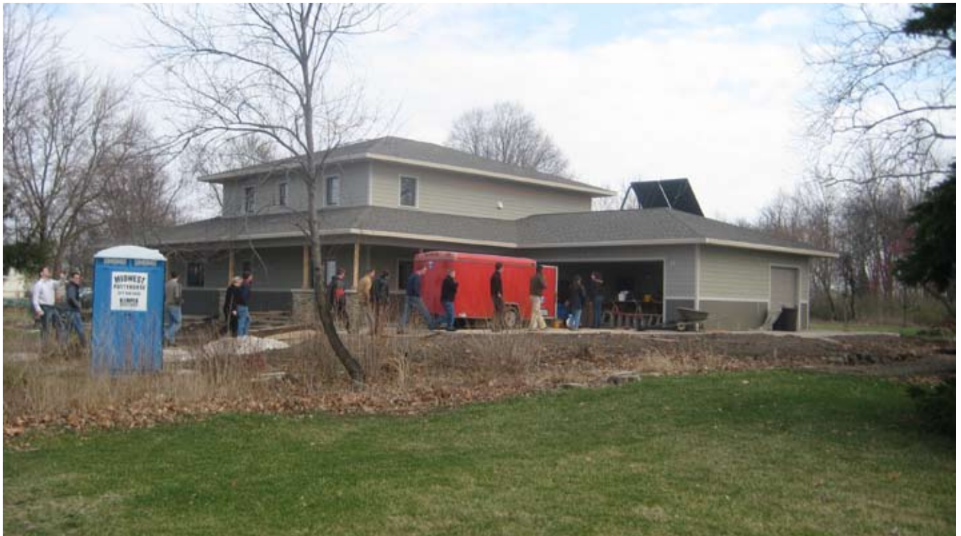
Image 3: Passive House in Urbana, IL: Notice the size and number of windows along the north and west sides, as well as the overhangs and north side porch, compact building shape and solar thermal system above the garage (Photo credit: Joe Gransee-Bowman).
