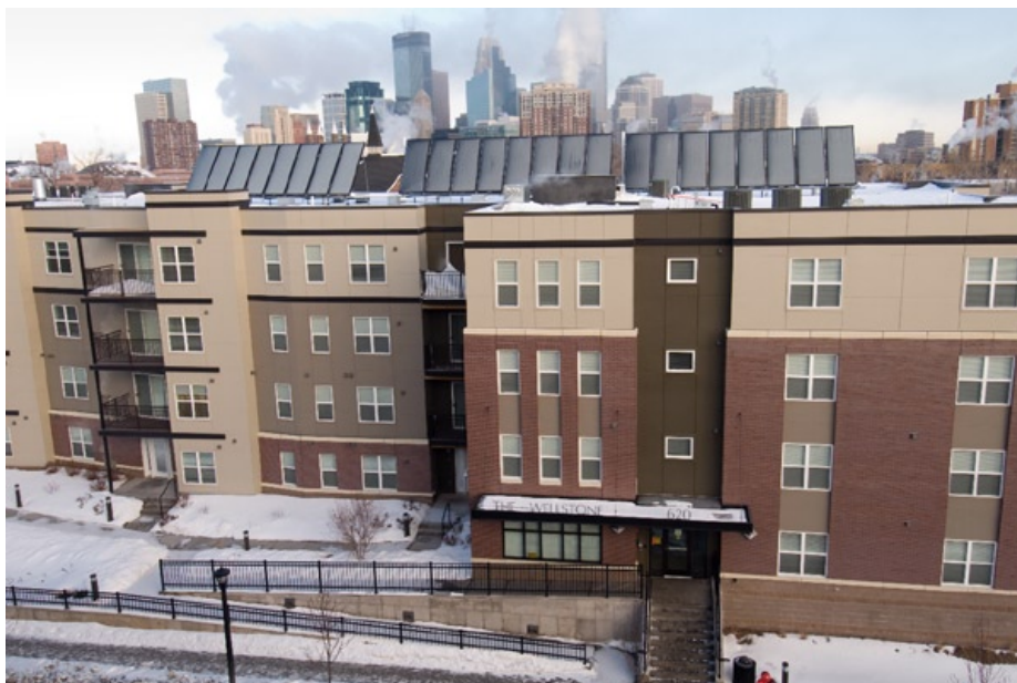
Solar Skies' Solar Thermal panels on the Wellstone Center in St. Paul, MN Photo Credit by Craig Tarr - Energy Concepts
