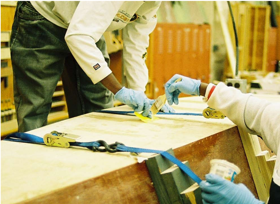
Filling screw holes after attaching the second side panel.
